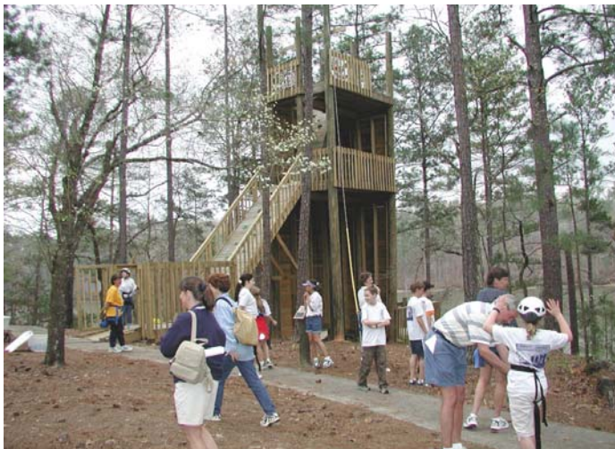
A full view of the tower.
